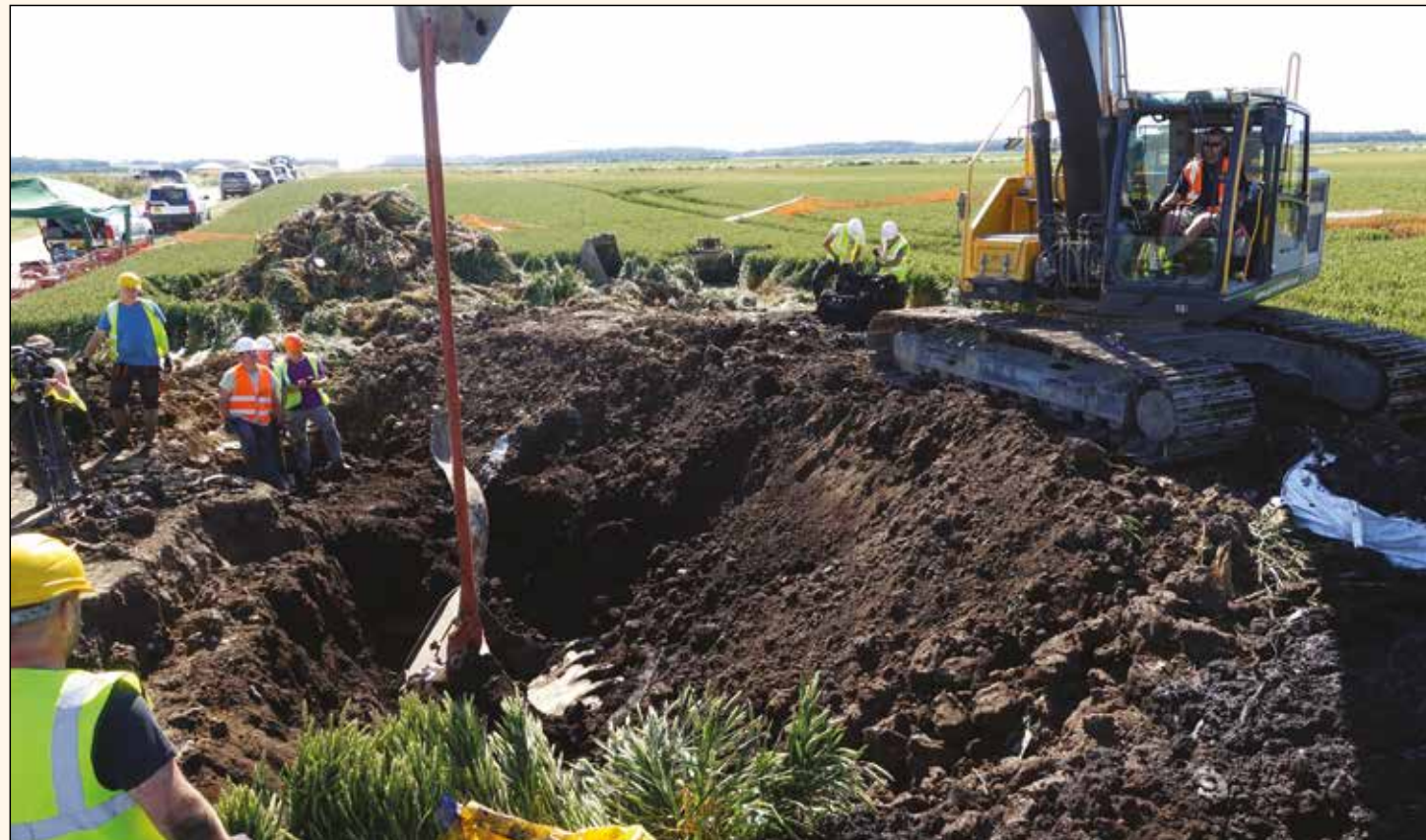
Left: This view of the propeller being lifted out of the hole shows the comparatively shallow depth that the wreckage was found at and the extent of the excavations. The dig took place in a huge open expanse of Lincolnshire 'prairie' on a very hot and windy day in June 2018.
